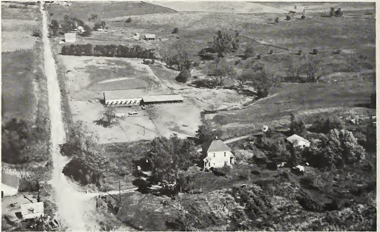
Before project: Erosion, sediment, and flooding are products of unprotected watersheds.
